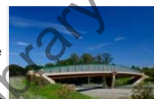
ET Bridge over the Maine Turnpike
